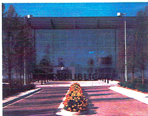
10,000 Square feet of Republic's own Heat Mirror™ windows were installed on the face of its award-winning plant to reduce energy use on a grand scale.
