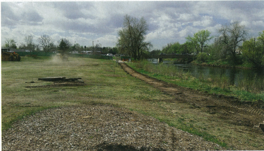
Pasquinel's Landing at the first stage of construction
