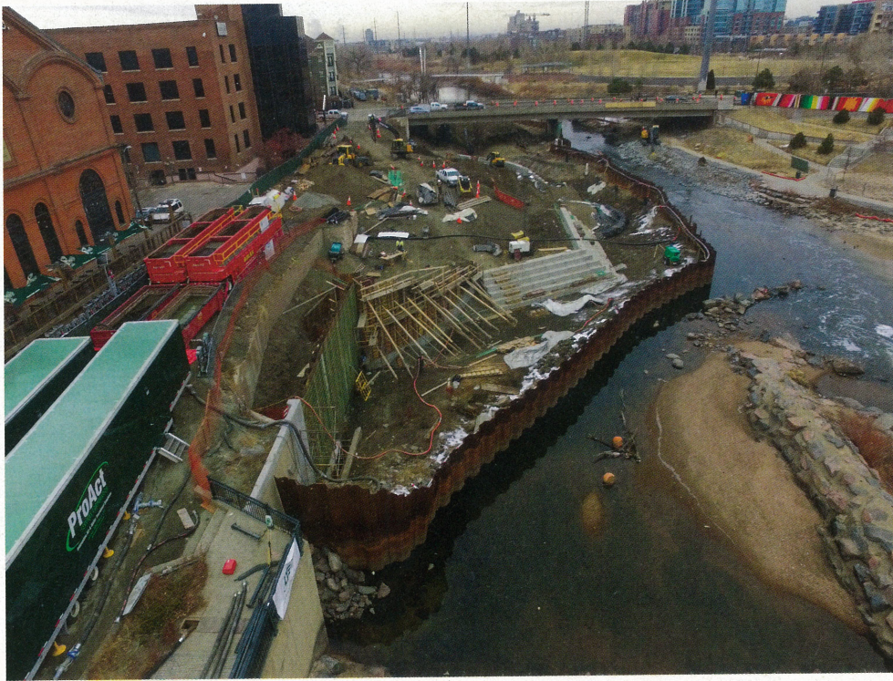
Removing coal tar from the South Platte at Confluence Park
